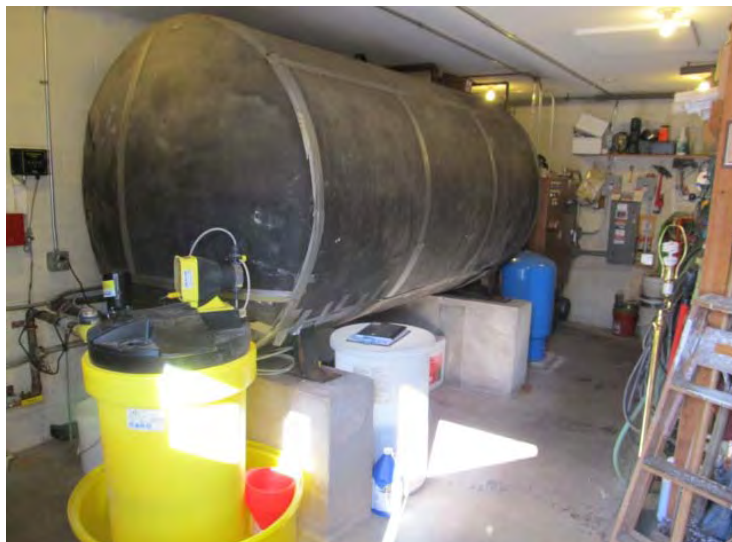
View of select components of well water system - Storage tank (in black), expansion tank (in blue), pressure booster pumps and control panel in background
