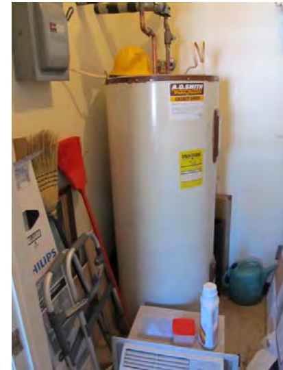
Electric domestic hot water tank for common areas – Serviceable but beyond expected useful service life
