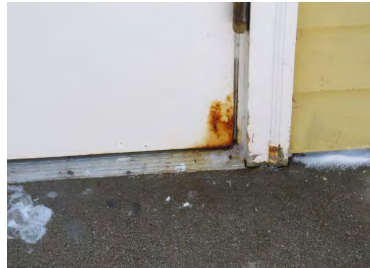
Rust damage noted on entry door to community space
