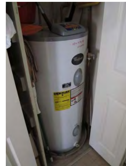
Each unit has its own electric domestic hot water tank
