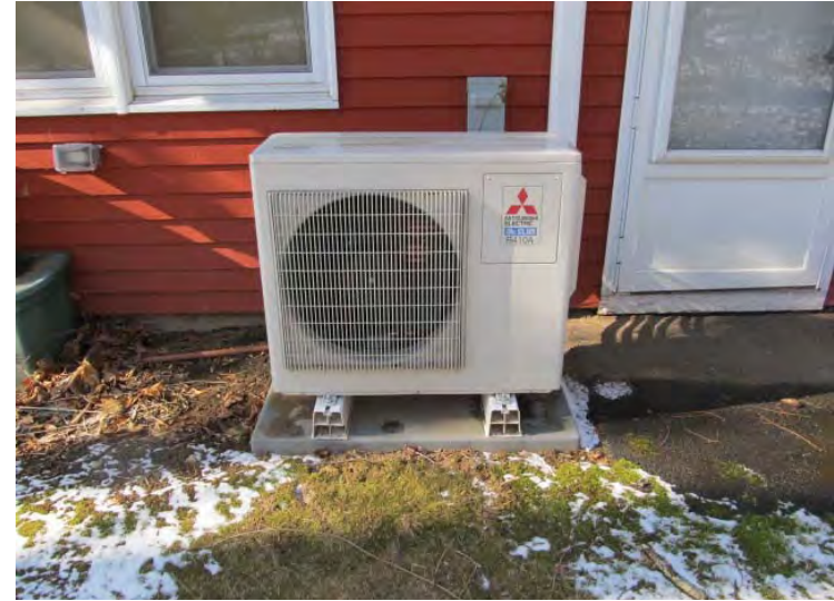
Typical, recently installed, exterior condenser for in-unit ductless mini-split heat pump system
