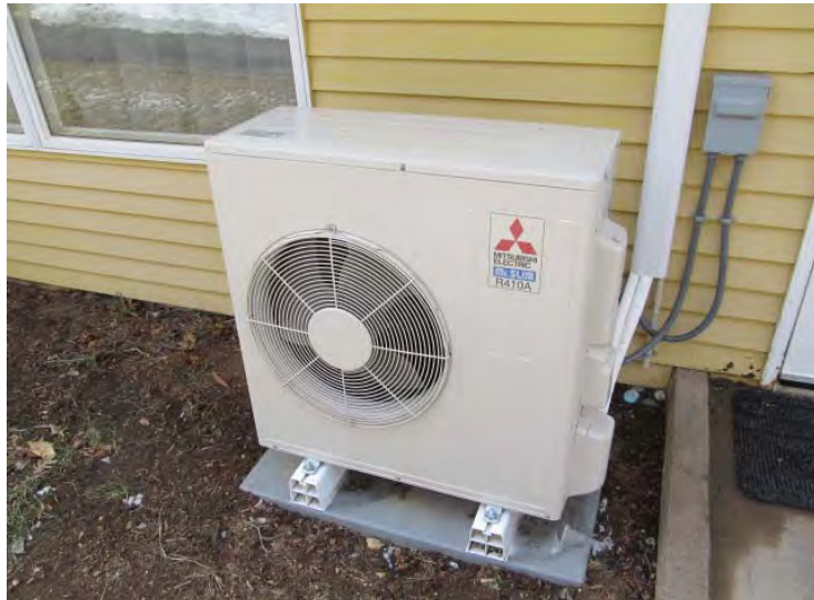
Exterior condenser for recently installed heat pump system at community spaces
