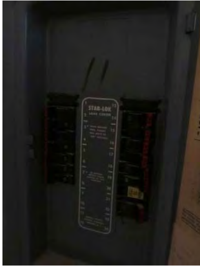
Unit electrical load centers feature Stab-Lok circuit breaker panels by Federal Pacific
