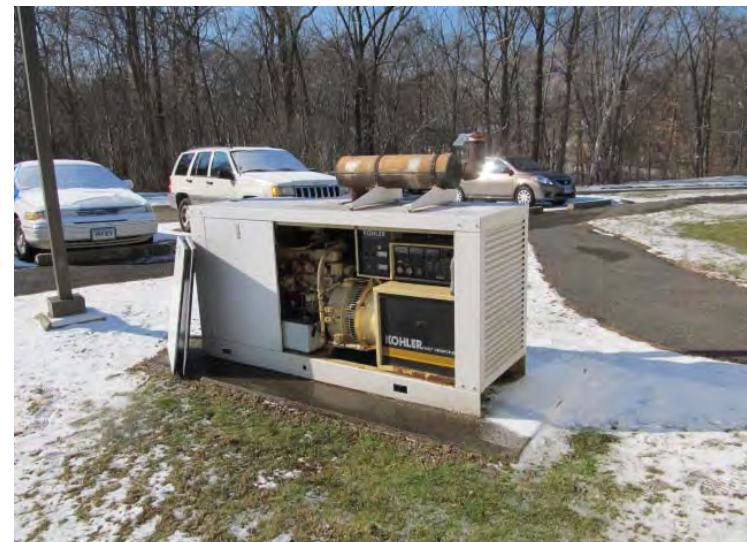
Propane-fired emergency generator – Serviceable but nearing end of expected useful service life
