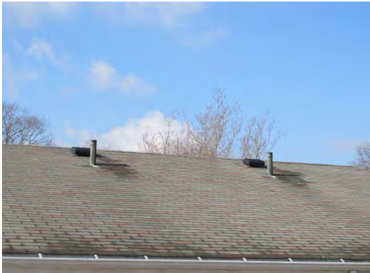
Roof shingles are nearing the end of their expected useful service lives
